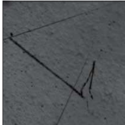
Inspection for Defects
